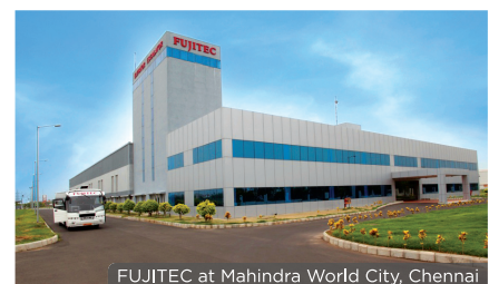
FUJITEC at Mahindra World City, Chennai
